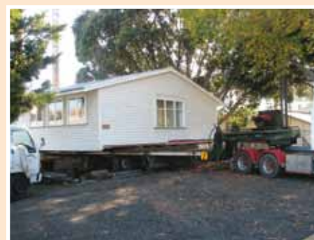
Tauranga Hospital's former HIA (Health in Ageing) building is transported to the Whakatane Hospital campus.
