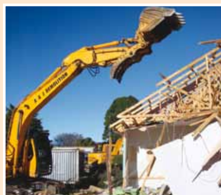
The Maternity building is demolished
